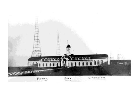
Fifty years have passed since the building of this great station, and (at least to my knowledge) none larger has been built. The 1000 kW CW transmitter at "Jim Creek" in Washington state is, however, of equal power if not in size and outlay. The duplicate 1000 kW arc transmitters at Lafayette weighed 83 tons each, and the huge antenna was 408 meters wide by 1200 meters long! Eight 820-foot towers supported the huge L antenna, directional toward Annapolis, Md—"NAA."<sup>1</sup>
