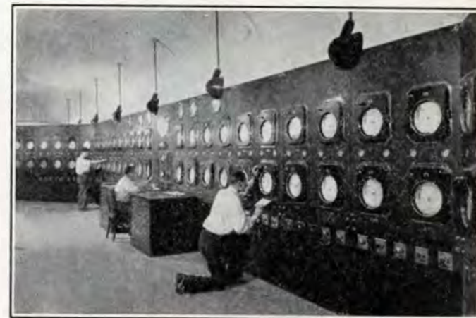
Control panel for large air conditioning plant in NBC's section of Radio City
