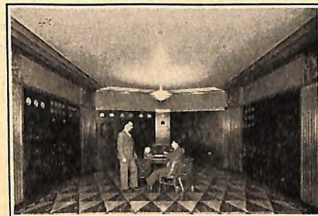
Main transmitter room of station WEAJ. Modulating and frequency control at left, 50KW amplifier in center, power control equipment at right
