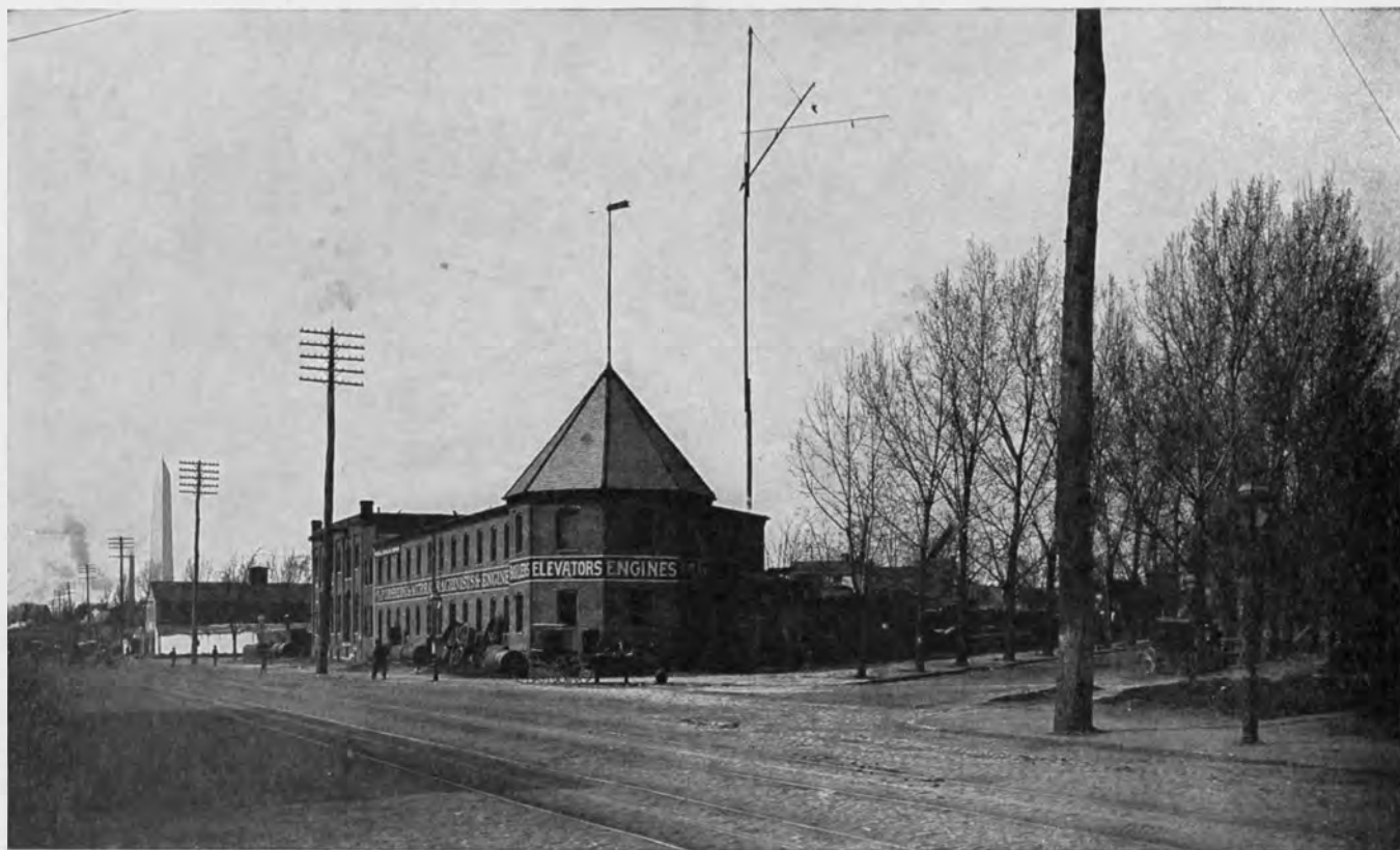
FESSENDEN WIRELESS TELEGRAPH STATION.
