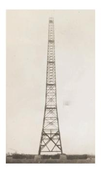
The tower photo comes from the Stanford University archives, "The Birth of Radar! 247 ft Self Supporting Wooden Tower supporting Six pairs of Double Dipole Antennas. Designed & Built by C. F. Elwell 07/08 (77 built in England)." typed on back. "247' S. S. wooden towers for British Radar - 1936. 66 off - designed, contracted by C. F. Elwell" written on back. Photo ID: 15067 Folder Title: Elwell, Cyril F. -- instruments -- #2 RADAR Tower photo [.]
